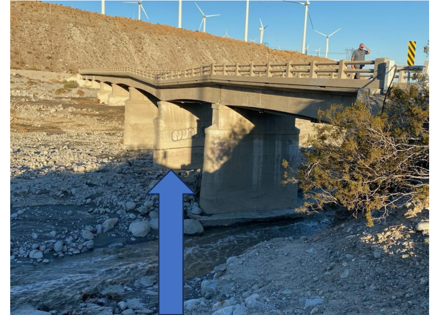
Whitewater Rd Bridge Pier scoured and dropped
