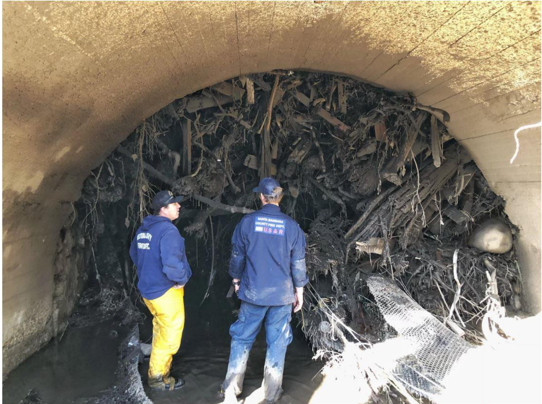
Bridge at creek in Montecito filled with debris from the January 9 deadly rains and mudflow (Photo by Blake Herman/SB County Fire via SBC Fire Info Twitter)
