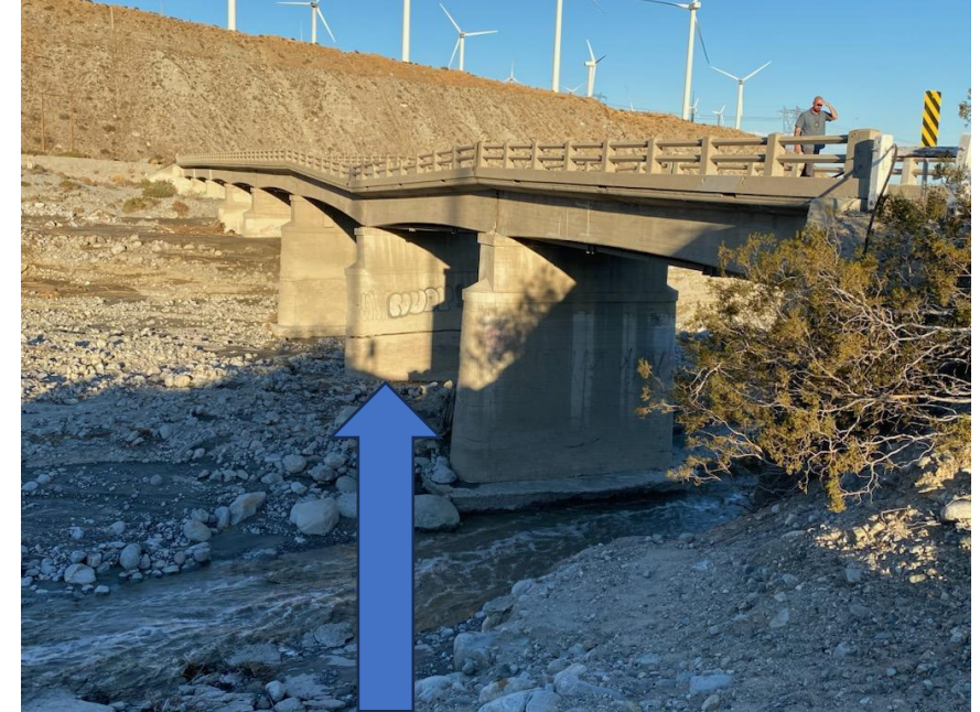
Whitewater Rd Bridge Pier scoured and dropped
