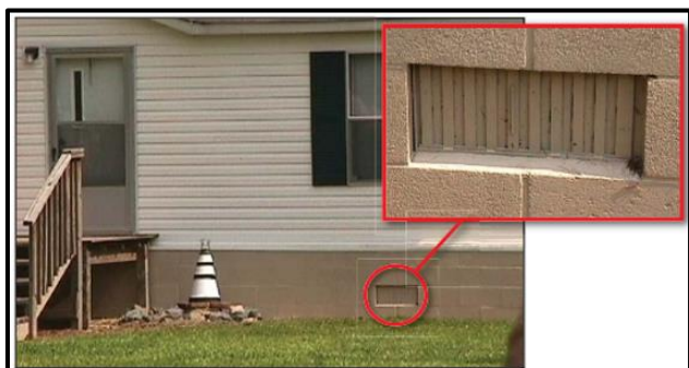
Unacceptable flood vents. Flood vents must remain open.
