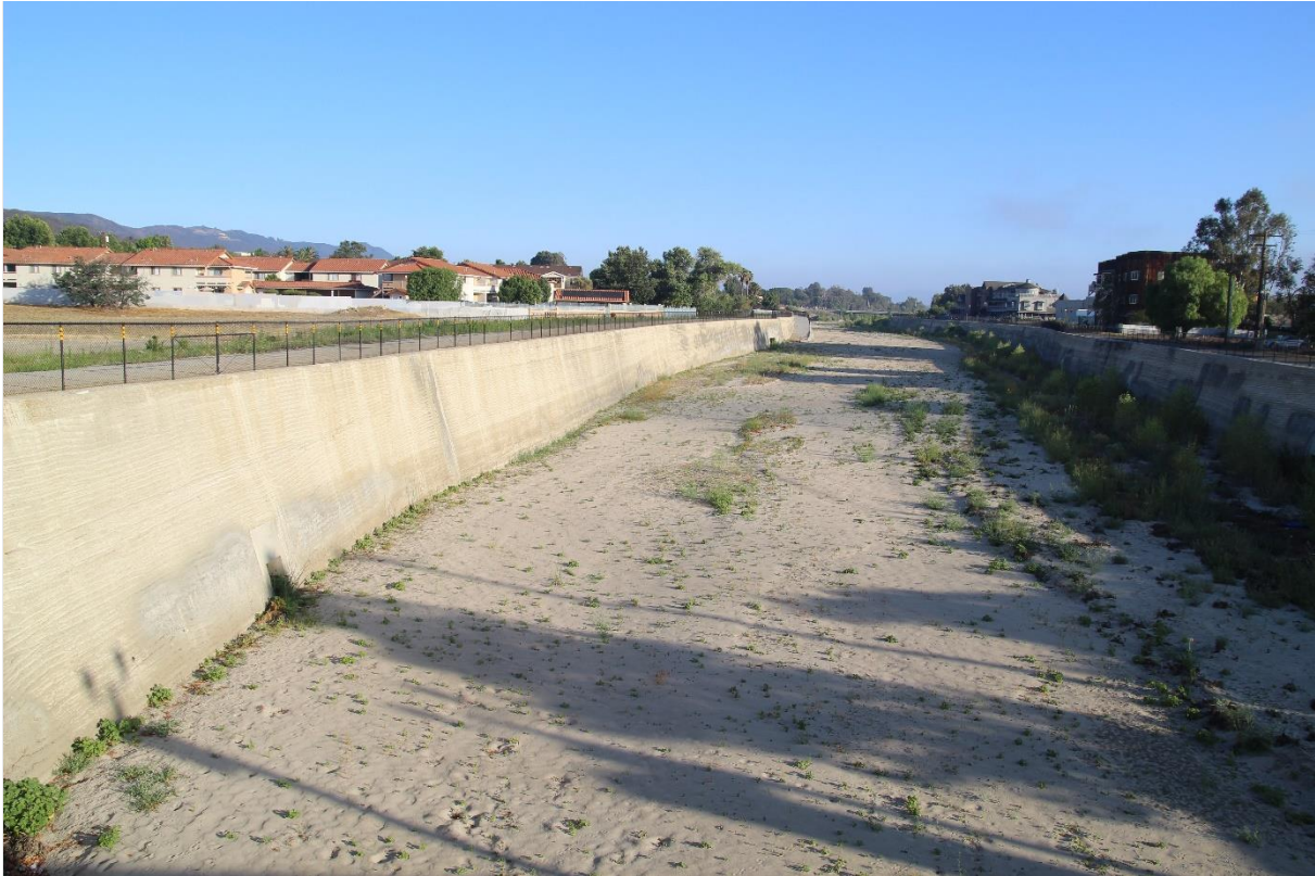
Figure 8.6: Soil Cement Side Slopes
