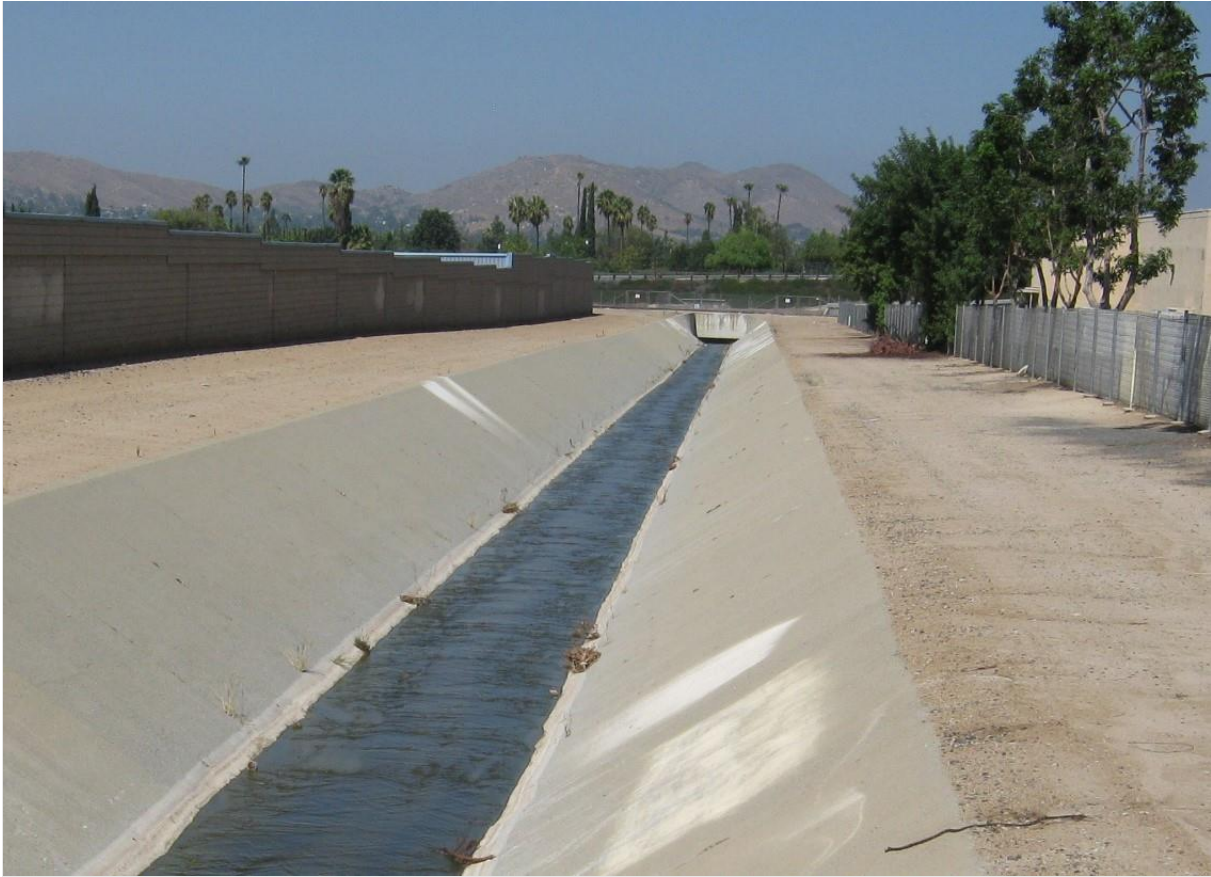
Figure 8.4: Concrete Lined Channel
