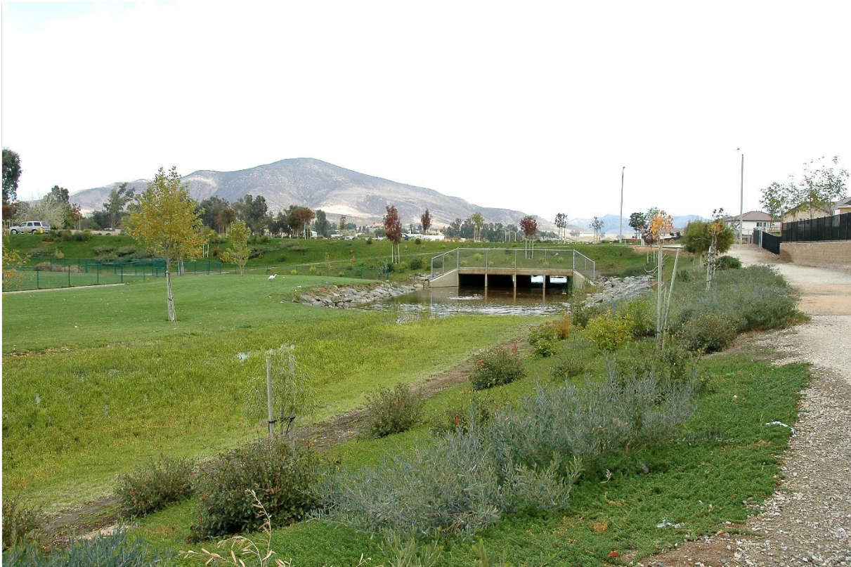
Figure 8.3: Grass Lined Channel
