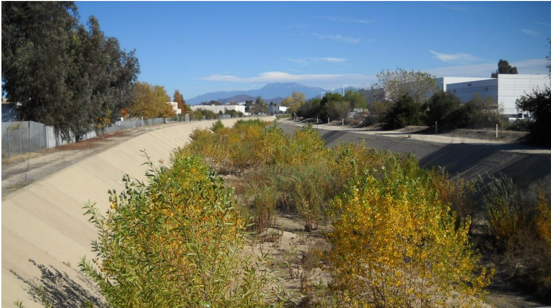
Figure 8.7: Soft Bottom, Bank Lined Channel
