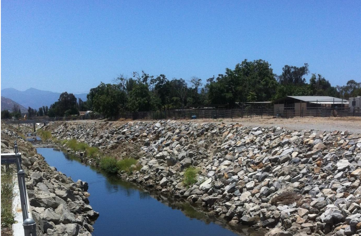
Figure 8.5: Rock Lined Channel
