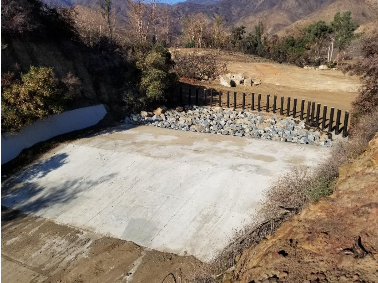
Figure 11.3: Debris Posts Upstream of Spillway
