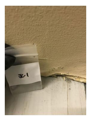
Picture 3: Ceiling joint compound was determined to be ACM by CAC
