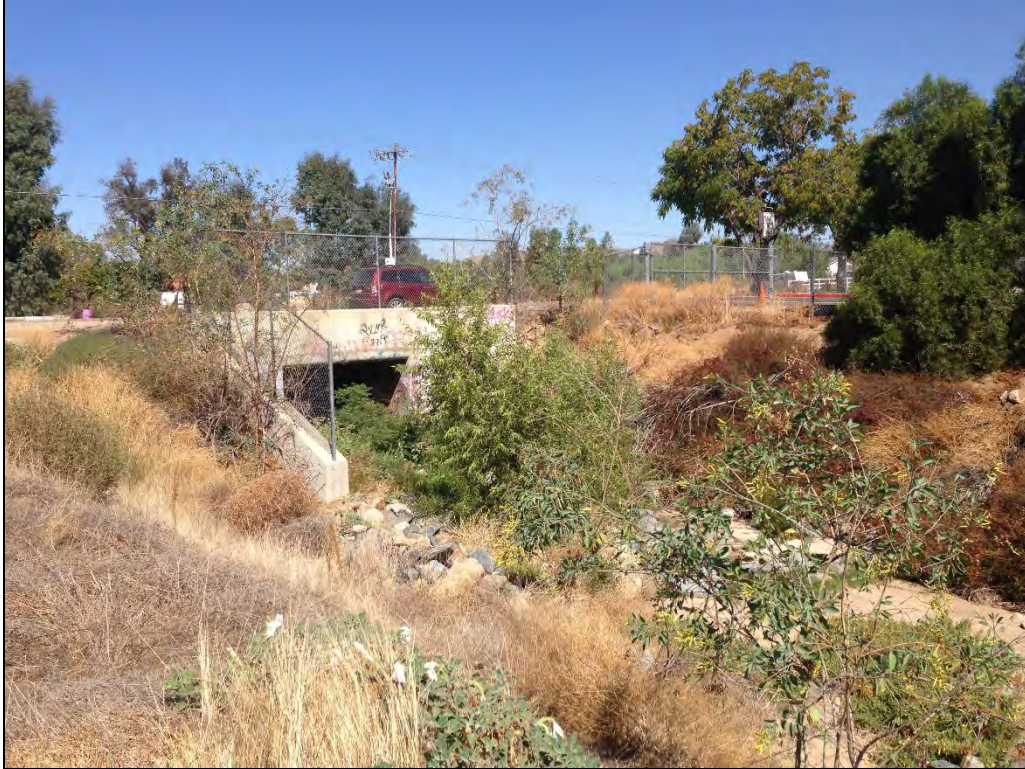
Photo 15. Existing ephemeral drainage crossing at Central Avenue
