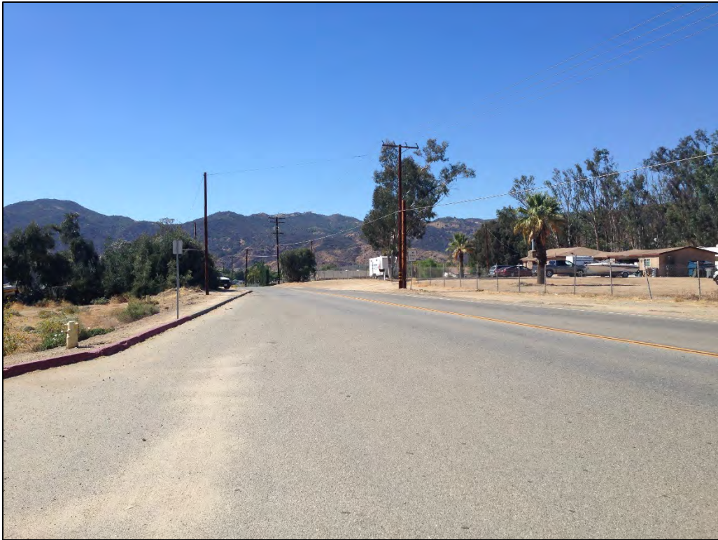
Photo 14. Central Avenue looking south, southern portion of the proposed Lateral C Main Line
