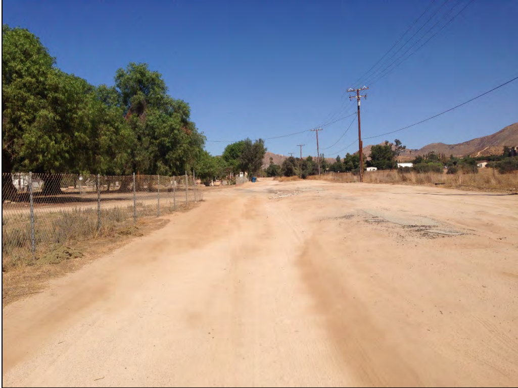
Photo 9. White Street looking north, central portion of proposed Lateral C Main Line
