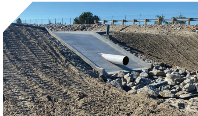
Bautista Basin Channel Recharge Basin expansion
