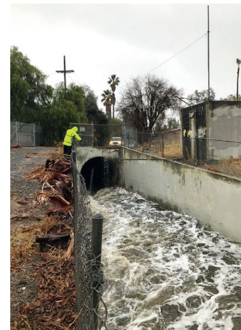
Sampling at Magnolia Center outfall
