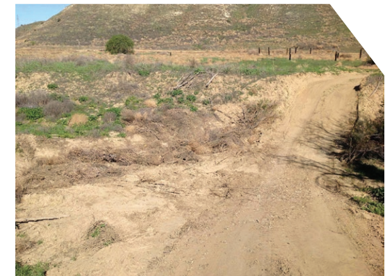
Before: Impact to the natural drainage within Aliso Creek
