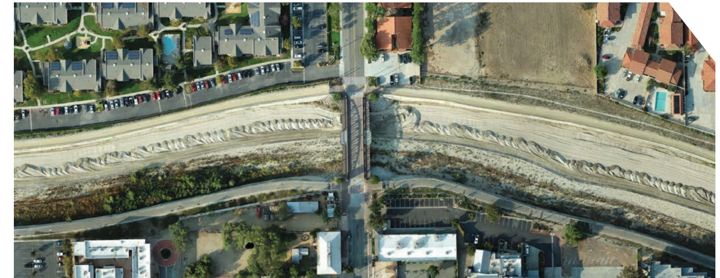
Murrieta Creek in Old Town Temecula Phases 1 and 2A. Open to the public for pedestrian, bicycle and equestrian use.
