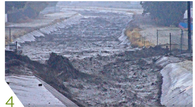
Noble Creek debris flow 12/24/2021 - 7:19am
