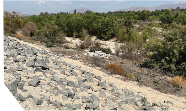
Santa Ana River levee
